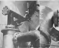
THESE ARE the close-up, intimate views of a production facility. In this case it is the Spent Acid Recovery Plant. ABOVE is part of a gas scrubbing tower and in the center and at right are piping which sport bulky insulation.
